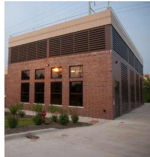
Generators Enclosed in Building
