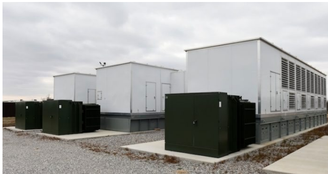
Larger Generator Units (2MW each)
